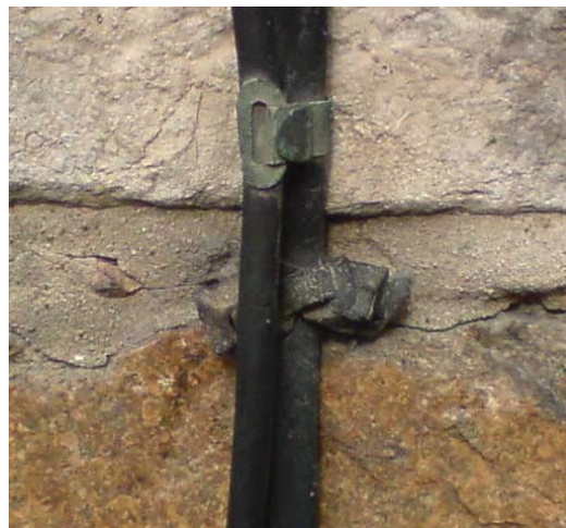
Fig 3. Cable showing iron/lead clip and buckle clip
